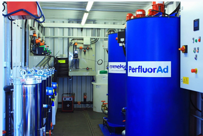
Mobile PerfluorAd Treatment Plant (Constructed in 20' Container)
